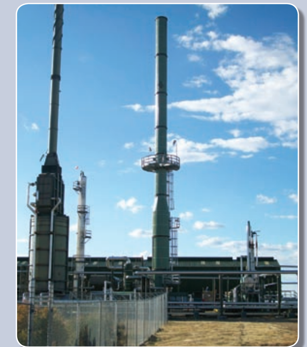
SRU tail gas incinerator designed for use in cold temperature climate.
